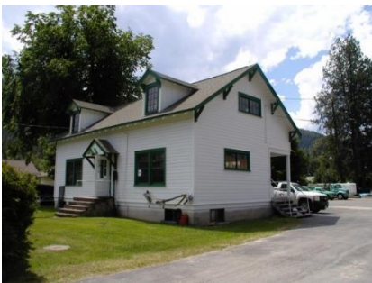
The remodeled Superior building in 2012. There is also a substantial addition in the back which is not visible in this photo.
