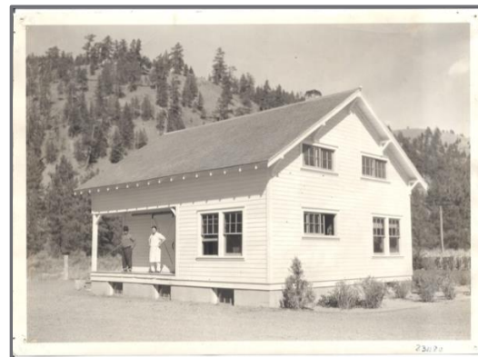
Bonita Ranger Station combination building 1930s. The remodeled and deserted building can be seen off the Rock Creek exit off Interstate 90 towards the end of the north frontage road.
