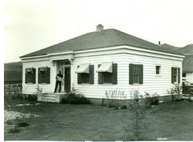
The Plains Ranger Station combination building, probably in the 1930s.
