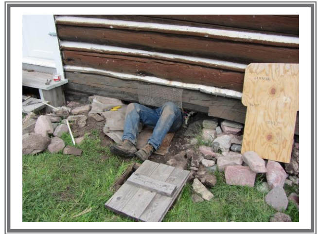
Backcountry plumber at work
