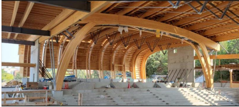
Fig. 1 – University of Idaho's new arena under construction.
