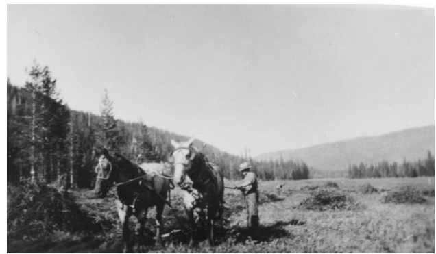
Horse team used during construction of the Fish Creek Airfield in 1933 or 1934.
