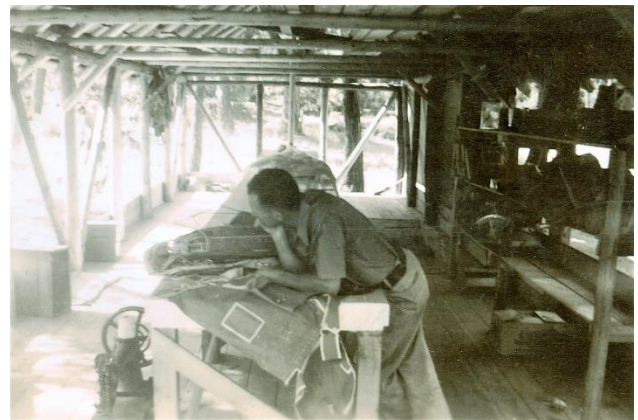
First parachute loft built by the 1940 crew at Moose Creek Ranger Station in July. Chutes were stored on shelves at right. Note sewing machine and long packing table. Frank made the original static line design on this table in July 1940, Nez Perce National Forest. Alexander, James A. "Smokey" photo from the National Museum of Forest Service History Collection.
