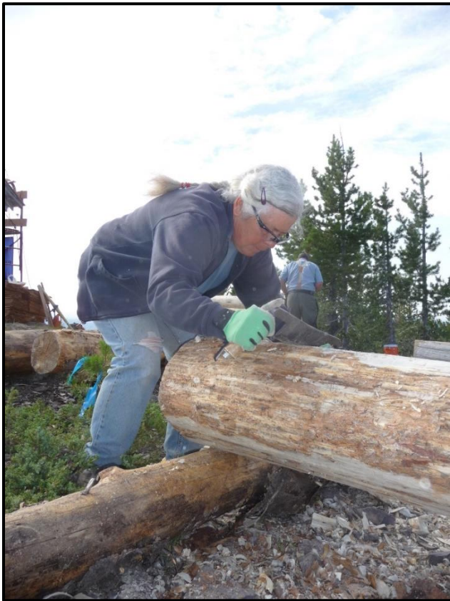
Vicky peeling logs. Big Hole Lookout Pit Project, 2016.
