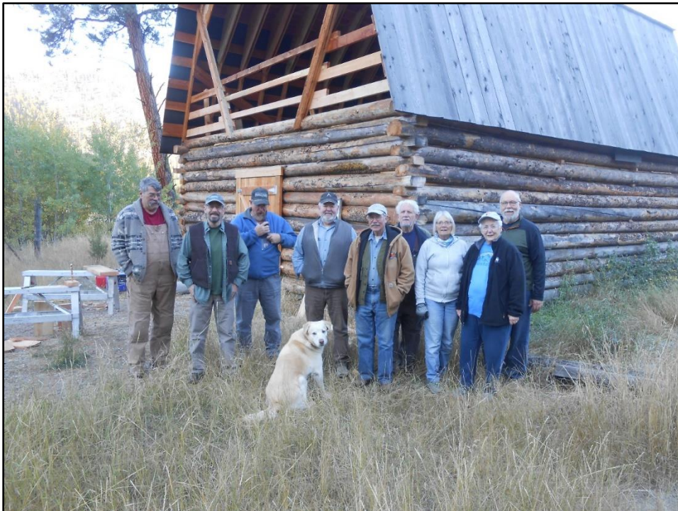
Friends at the newly re-constructed barn at Morgan-Chase Homestead, Granite County, Lolo National Forest.
