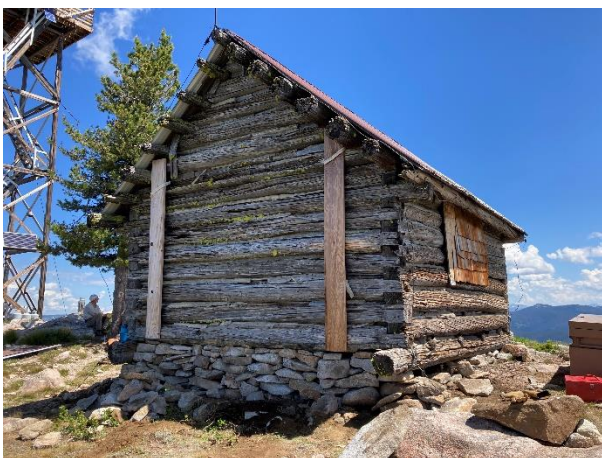
The cabin before preservation work started.
