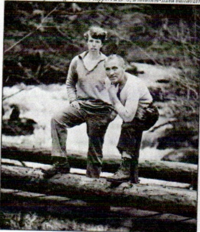
Astride "Penny's bridge"; it can support a D-6, a medium-sized bulldozer.
